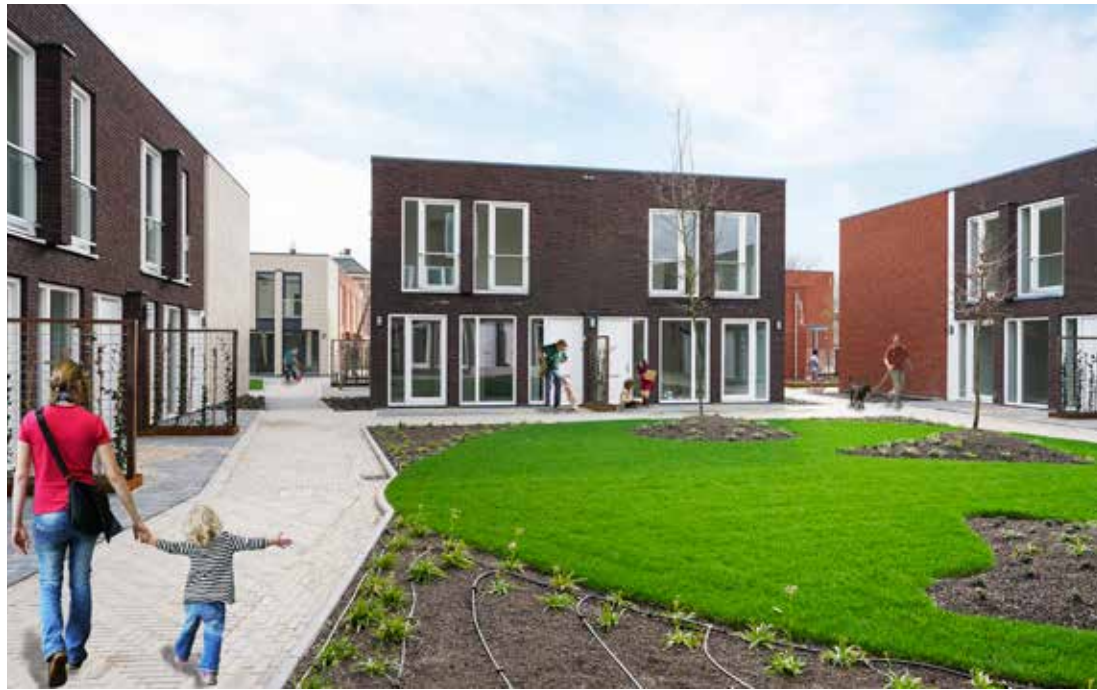
Vormen Fabriek Affordable Housing Tilburg, The Netherlands
