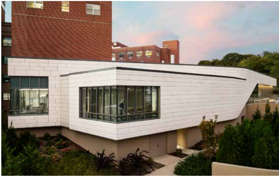
Northwell Health Huntington Hospital ED Huntington, NY
