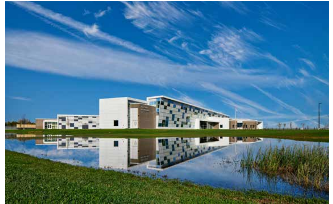
Illinois National Guard Army and Aviation Support Facility and Readiness Center - Kankakee Kankakee, IL
