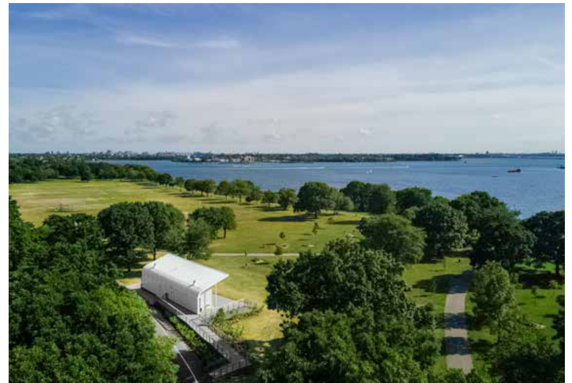
Ferry Point Park Comfort Station Bronx, NY
