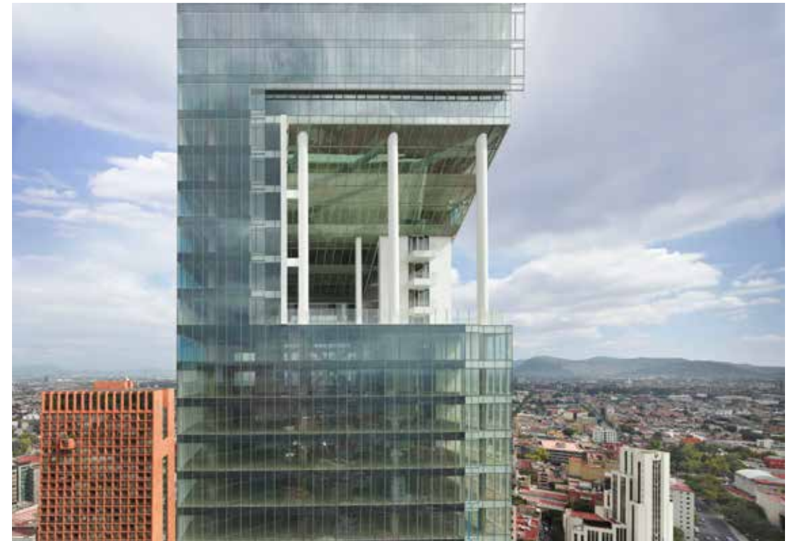
Torre Cuarzo on Reforma Mexico City, Mexico
