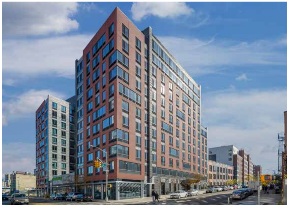
Navy Green Townhouses and Condos FX Fowle / Curtis+Ginsberg / Architecture in Formation Brooklyn, NY AFFORDABLE AND SUPPORTIVE HOUSING
