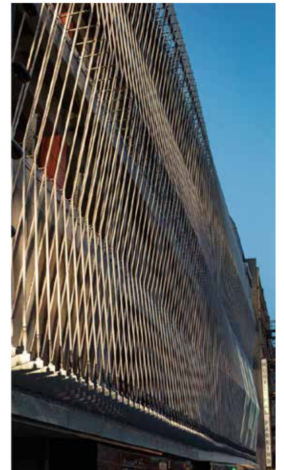
Delancey and Essex Municipal Parking Garage New York, NY
