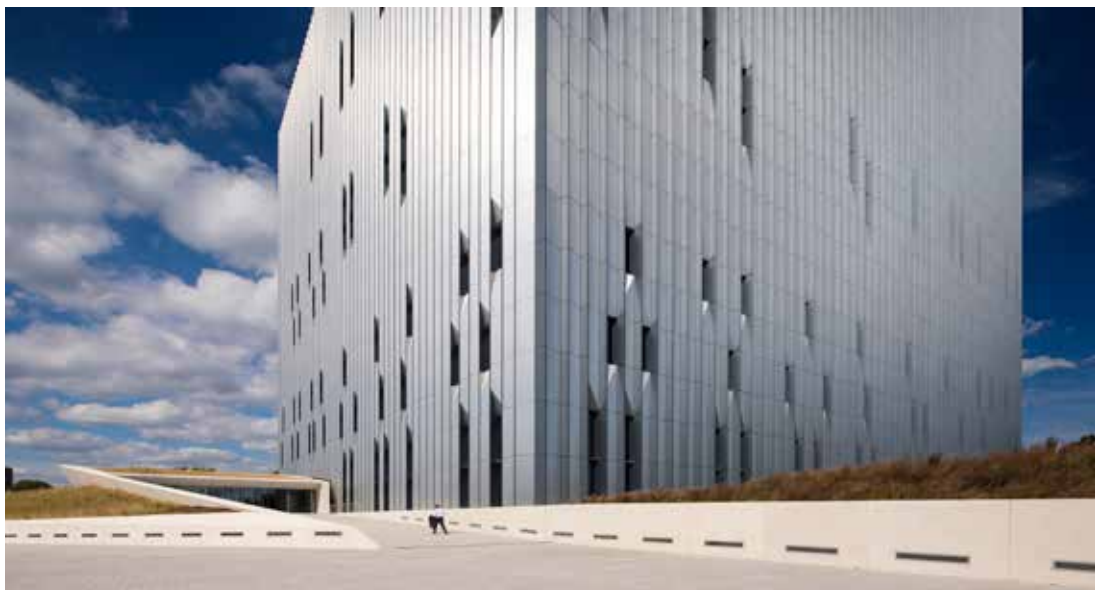
Public Safety Answering Center II Bronx, NY
