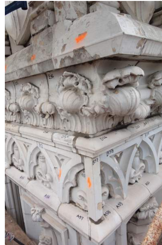
36 Gramercy Park East Exterior Rehabilitation New York, NY
