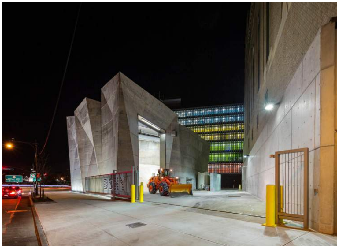
Manhattan District 1/2/5 Garages and Spring Street Salt Shed Dattner Architects New York, NY
